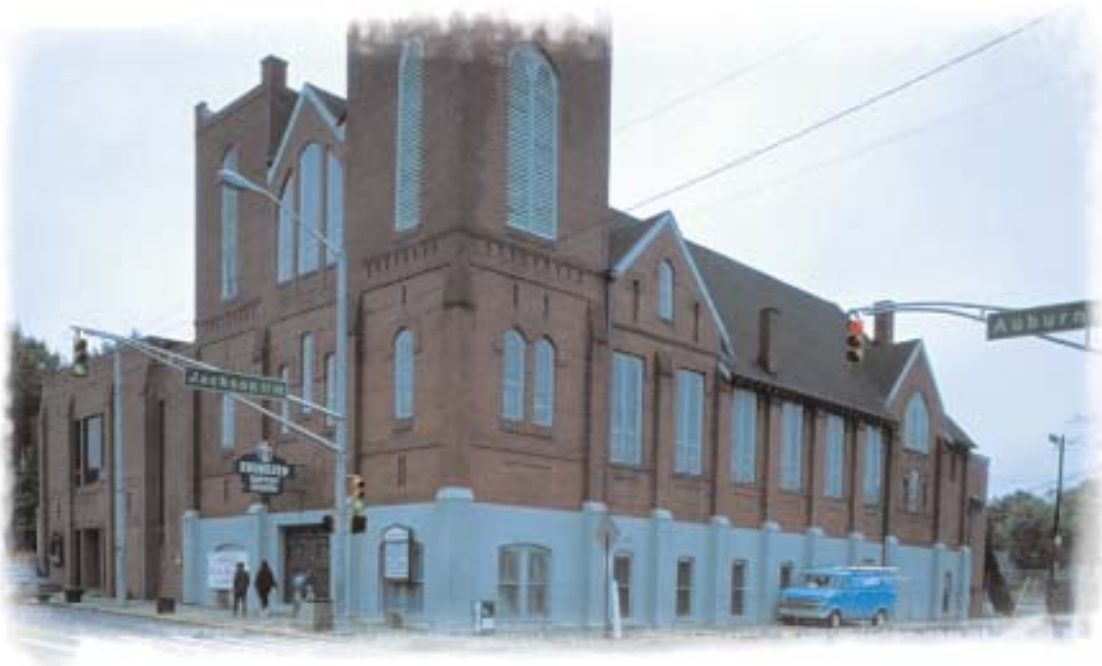
The Ebenezer Baptist Church at the Martin Luther King, Jr., National Historic Site in Georgia is slated to receive restoration funds in fiscal year 2005.
