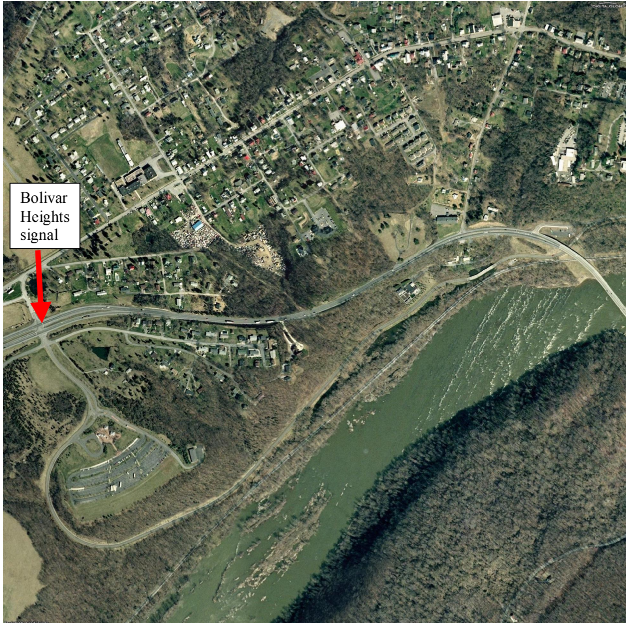
Figure 3: US 340 Four-Lane and Two-Lane Sections Including Bridge Over Shenandoah River
